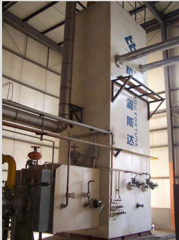
2000Nm 3 /h N 2 Liquefaction plant
